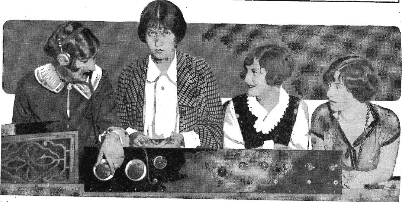
It is a far cry from the first one tube set in the experimental laboratories at Hunter College, New York, to the above photo. But, the girls have advanced to the super stage in the Radio division. They are shown assembling and testing a new eight tube super-heterodyne receiver with which they hope to "log" the coast regularly this winter.
